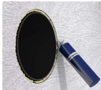
Fig. 5 Sealing the wall mounting pipe
