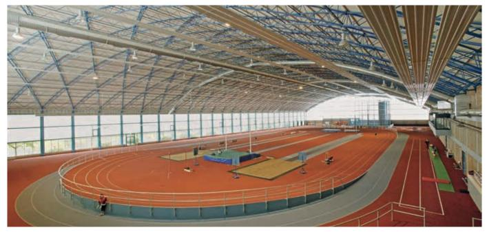
Because large glass front panels were used, the new heating system was required to guarantee year-round useability. The Zehnder ZIP radiant ceiling system met this challenge as well.
