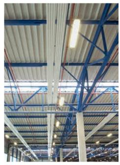
Emphasis is also placed on performance and efficiency in the area of climate-control technology, in the form of a Zehnder radiant ceiling system. 19 km of Zehnder ZIP radiant panels were installed.
