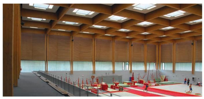
The 12,000 m<sup>2</sup> of the building have been fitted with Zehnder Reverse radiant ceiling panels which build a frame around the lighting. A total of 1836 m<sup>2</sup> blends perfectly into the idiosyncratic architecture.
