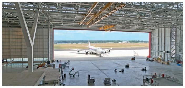
17,000 m<sup>2</sup> floor space, and a ceiling height of up to 42 m: an enormous challenge for Zehnder ZBN. The principle of thermal radiation takes full effect here, particularly considering that the heat is required mainly in the lower area of the hall.
