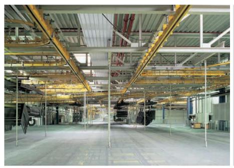
A total of 419 Zehnder radiant ceiling panel elements were installed in the new assembly halls. Their suspension was integrated without difficulty in the complex production lines of the fully automated paint shop.
