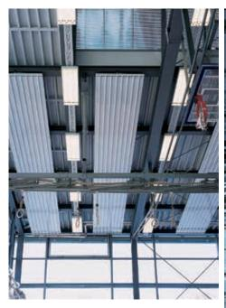
If it's sunny and the hall heats up rapidly, Zehnder radiant ceiling panels respond at speed. Thanks to their low water content, they match their thermal output to the external conditions in a flash. It's no wonder that Zehnder radiant ceiling panels, with their proven technology, rank amongst the most economical of any space heating system in the world.
