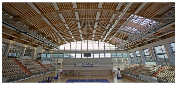
In order to heat the 5000 m<sup>2</sup> large hall evenly and efficiently, the decision was made to choose Zehnder ZBN. A total of 372 m<sup>2</sup> of perforated radiant panels for noise reduction were installed on the wooden structure which supports the roof of the hall.
