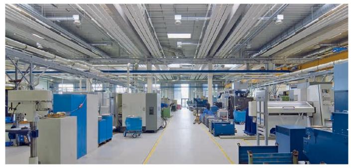
Zehnder ZIP or Zehnder Como products were utilised, depending on the individual department and its particular requirements. Ventilation outlets and lighting elements were integrated into the enclosed Zehnder Como ceiling sails.
