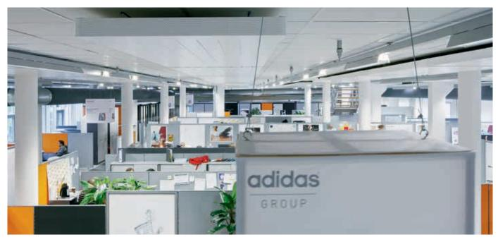
Areas where warm air collects in larger quantities must receive more cooling – and vice-versa. Thanks to the high radiation component of the flat panels, a comfortable indoor climate is achieved with high efficiency.
