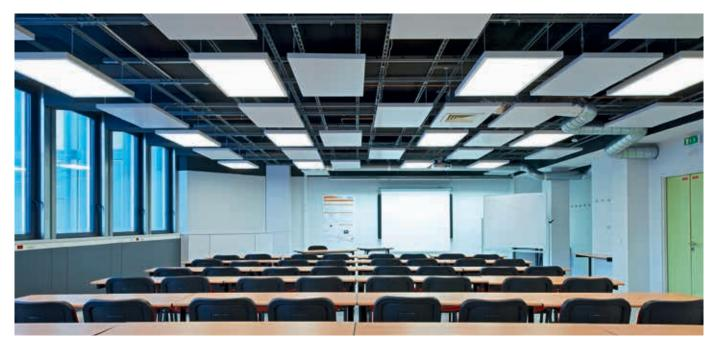
The building complex extends over a total area of 70,000 m<sup>2</sup>. 12,000 modules of the Zehnder Carboline radiant ceiling system were installed over 7275 m<sup>2</sup>.
